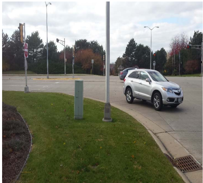
looking west from SE corner
