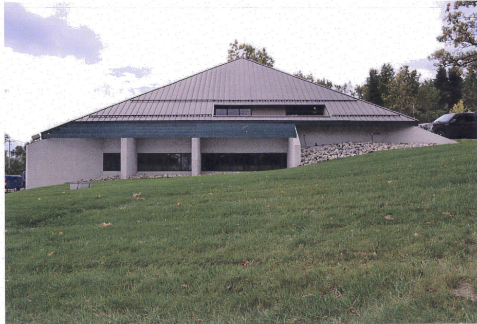
4 SD002 EXISTING NORTH ENTRANCE NOT TO SCALE
