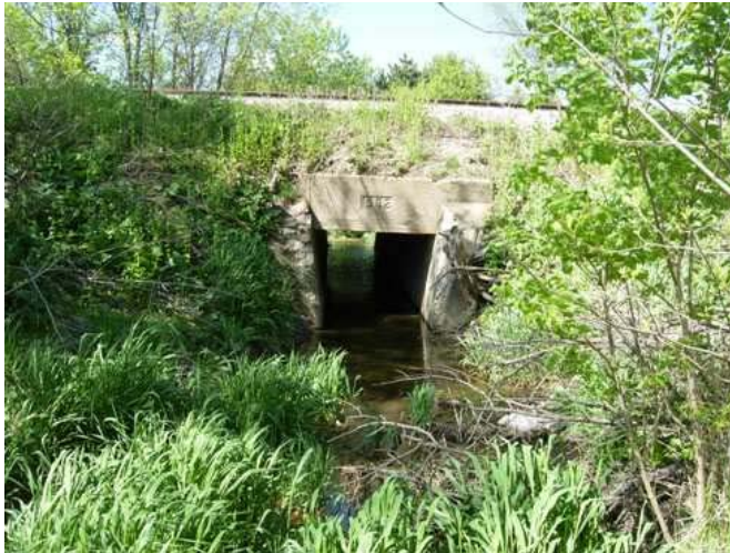
Figure 5 Downstream (south) end of railroad culvert
