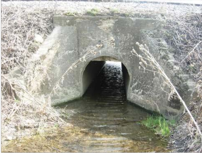
Figure 4 Upstream (north) end of railroad culvert
