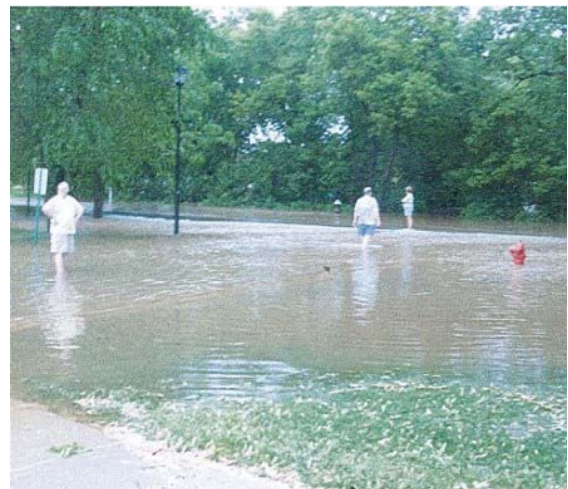
Figure 9 Floodwater overtopping Green Road (looking NW)
