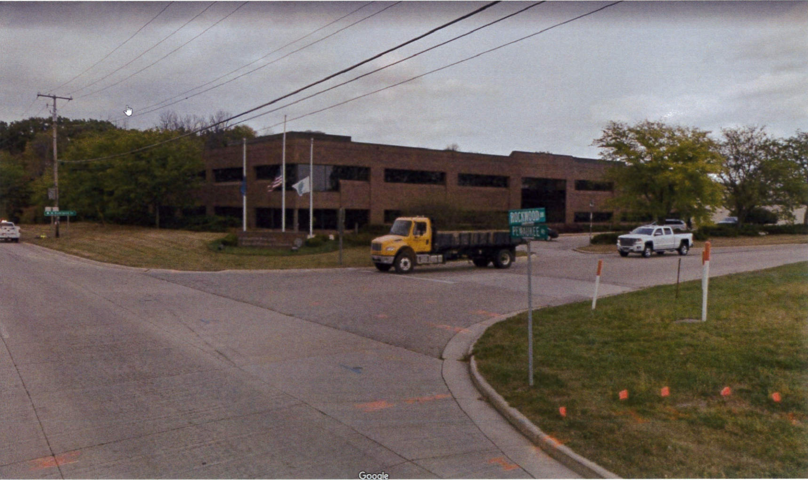
EXAMPLE OF ACCUMULATIVE ROOF SCREENS - STREET VIEW OF PEWAUKEE RD AND ROCKWOOD DRIVE - SEWRPC BUILDING
