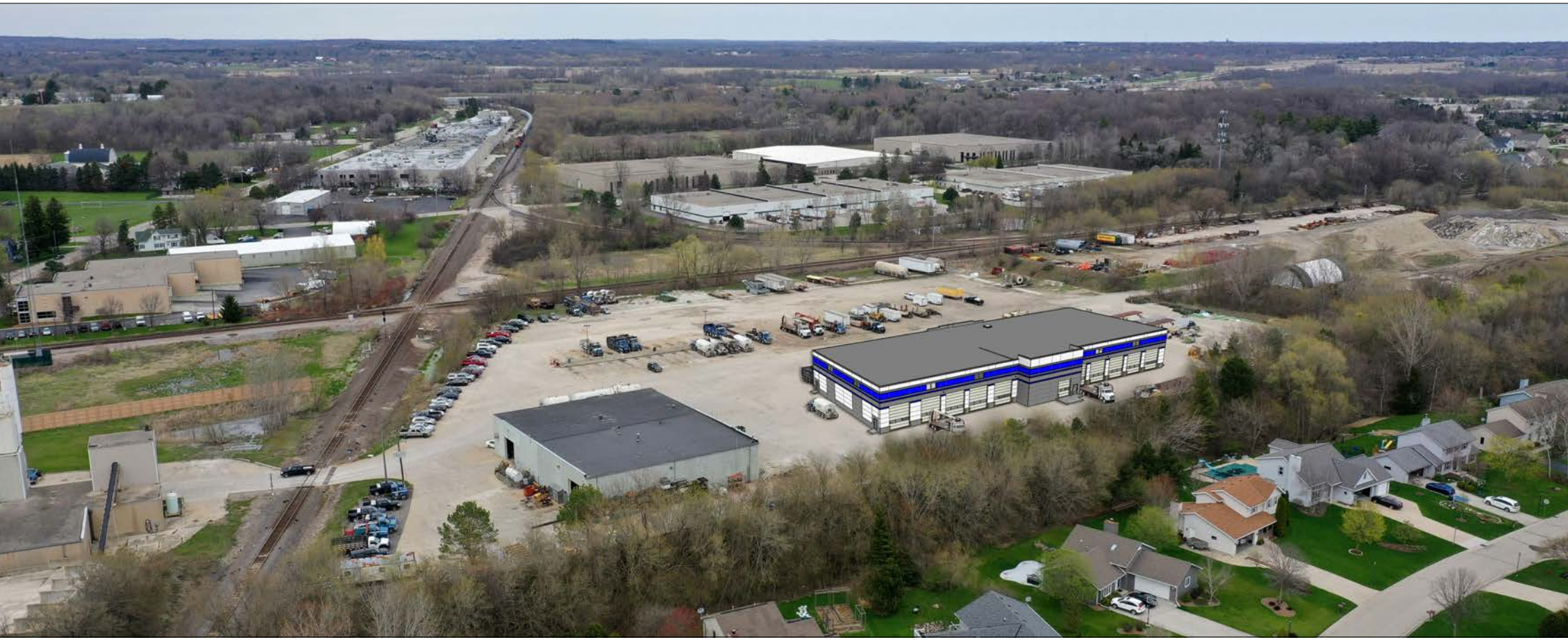
2 AERIAL VIEW - LOOKING NORTH / NORTH EAST NO SCALE
