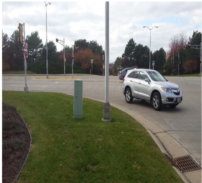
looking west from SE corner
