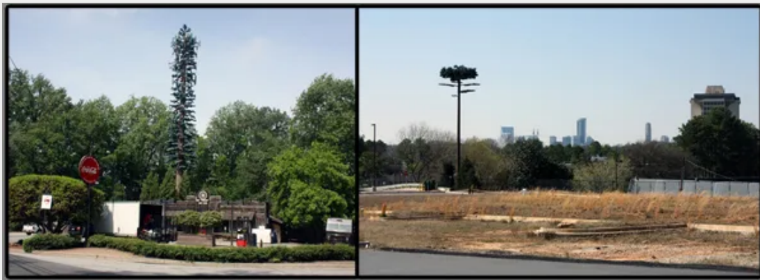
— Mt. Paran Road monopine (left) and monopine on North Druid Hills Road. Photos by David S. Rotenstein
