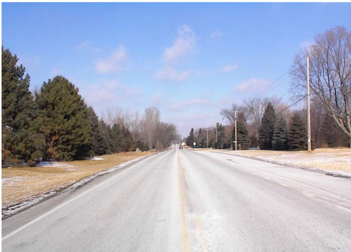
Looking north from Glenwood Lane
