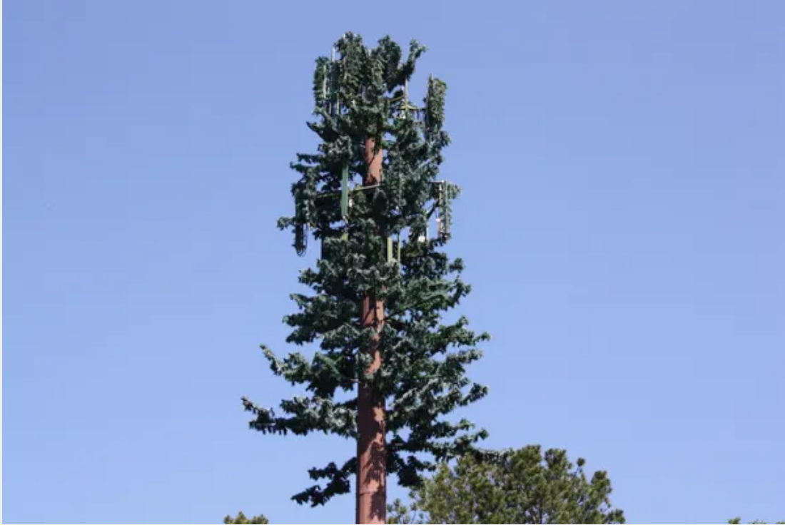
— Closeup of Morningside monopine showing antennas and fake branches. Photo by David Rotenstein.
