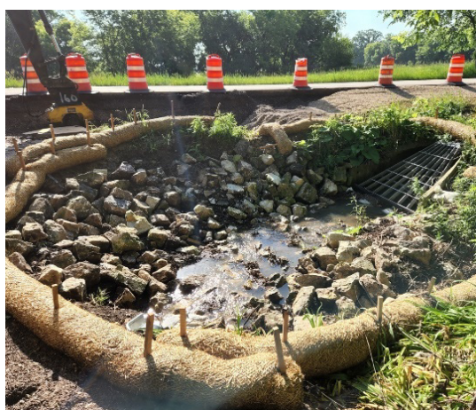
New culvert (left), erosion control (middle), and trench for new low flow storm pipe and structure (right).
