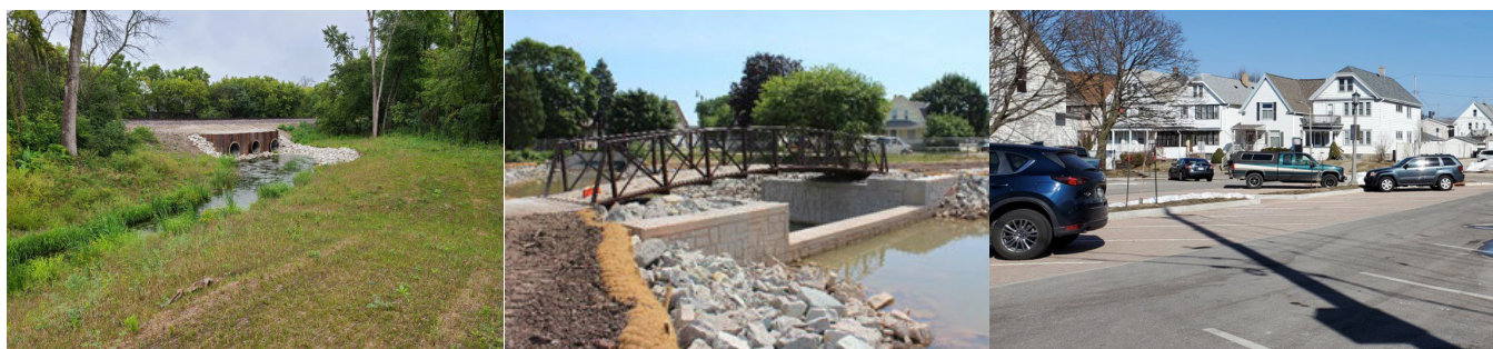
City of Pewaukee Emerald Acres project (left). City of Oshkosh South Park Design Project (center) City of West allis Parking Lots with Green Infrastructure (right).
