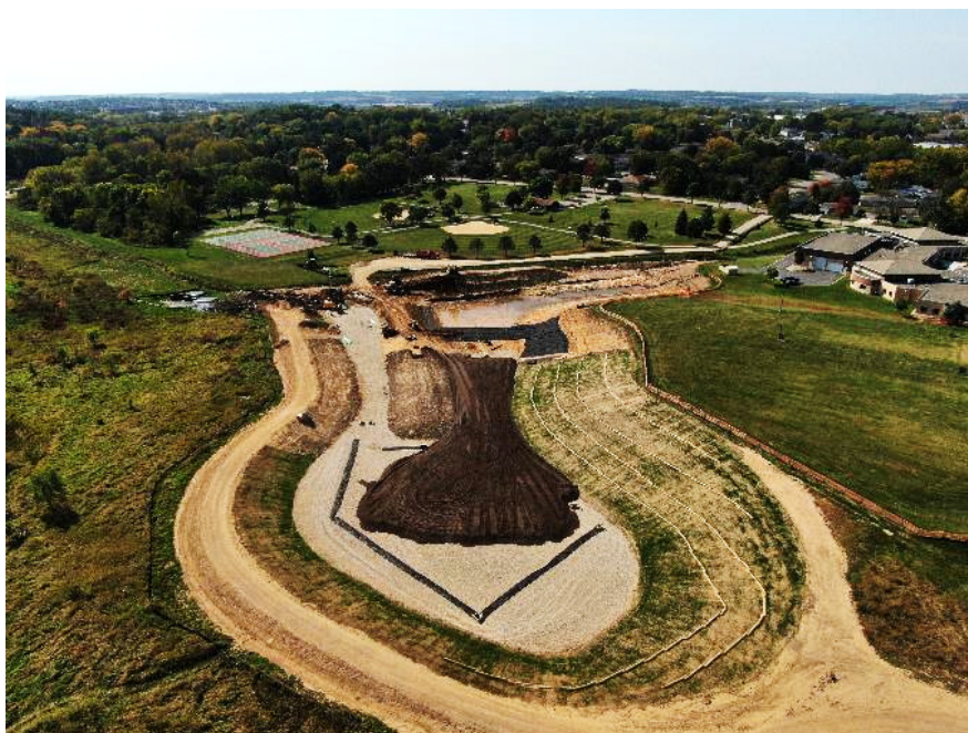
Left. Lincoln Street Storm water Management Facility under construction in September 2021. (Photo credit: City of Verona)
