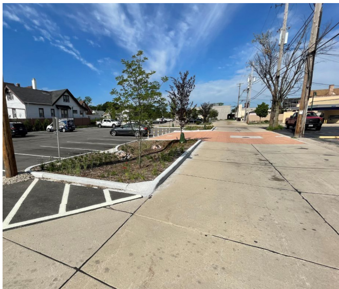
West Allis parking lot with two biofilters and permeable pavement (left). West Allis parking lot with permeable pavement and rain gardens (right).
