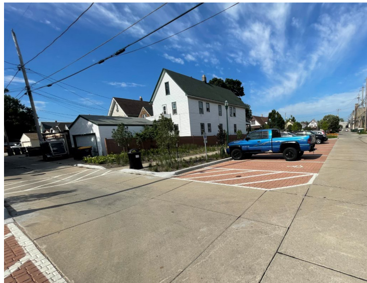
West Allis parking lot with two biofilters and permeable pavement (left). West Allis parking lot with permeable pavement and rain gardens (right).
