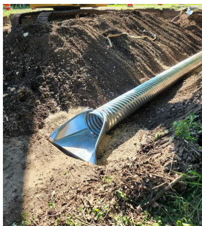
New culvert (left), erosion control (middle), and trench for new low flow storm pipe and structure (right).
