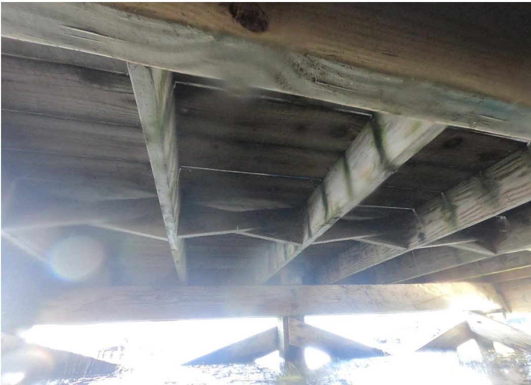
Typical underside view of West pier.
