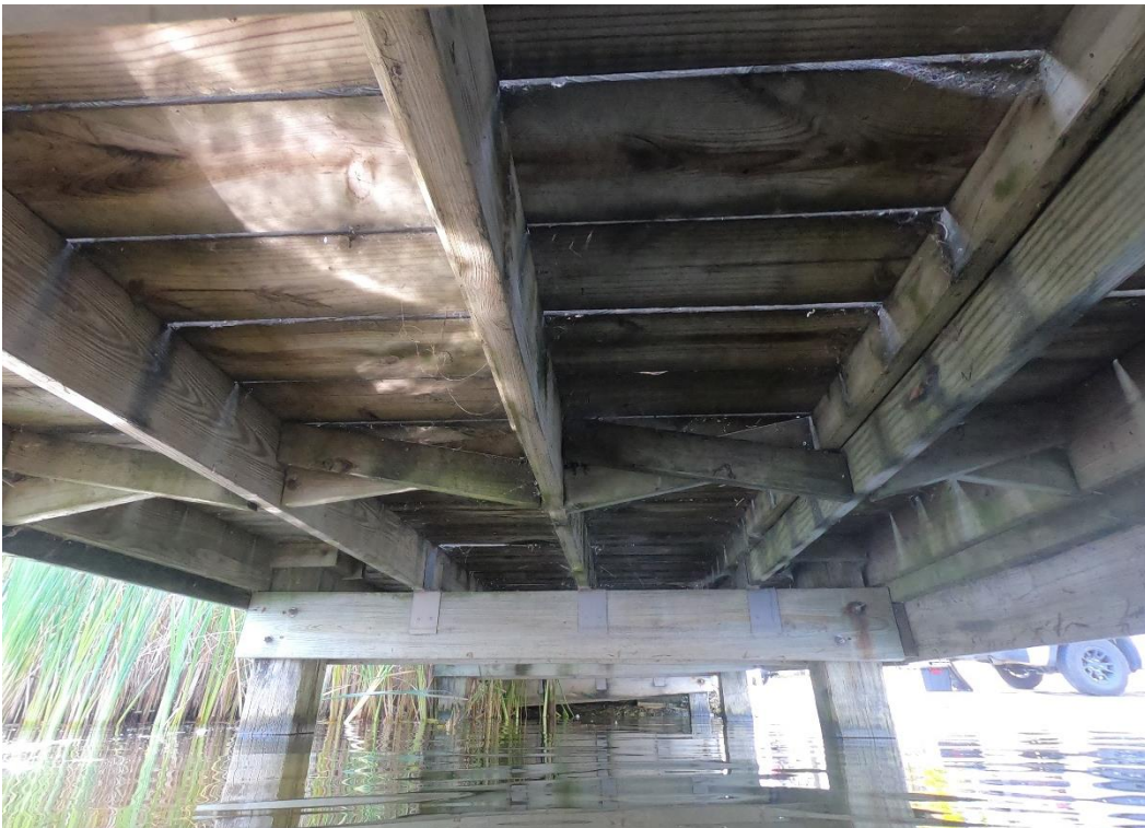
Typical underside view of East pier.
