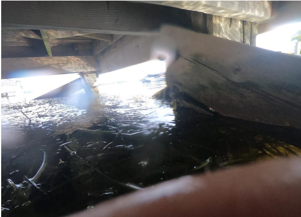
1 Column south of NE Corner of West pier with split cross brace on east edge.
