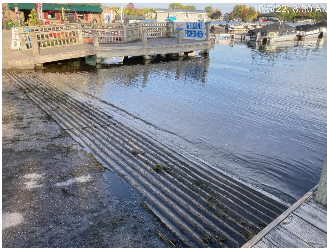
Overall view of corrugated concrete at top of boat launch.
