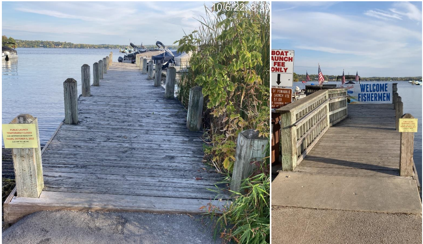
(Left) Overall view of East pier. (Right) Overall view of West pier.
