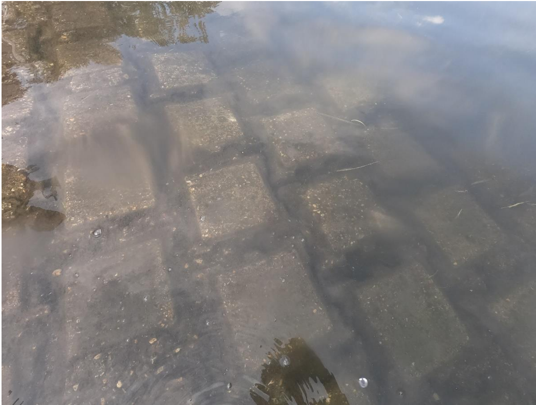
Typical view of the revetment mat at the start of the ramp.
