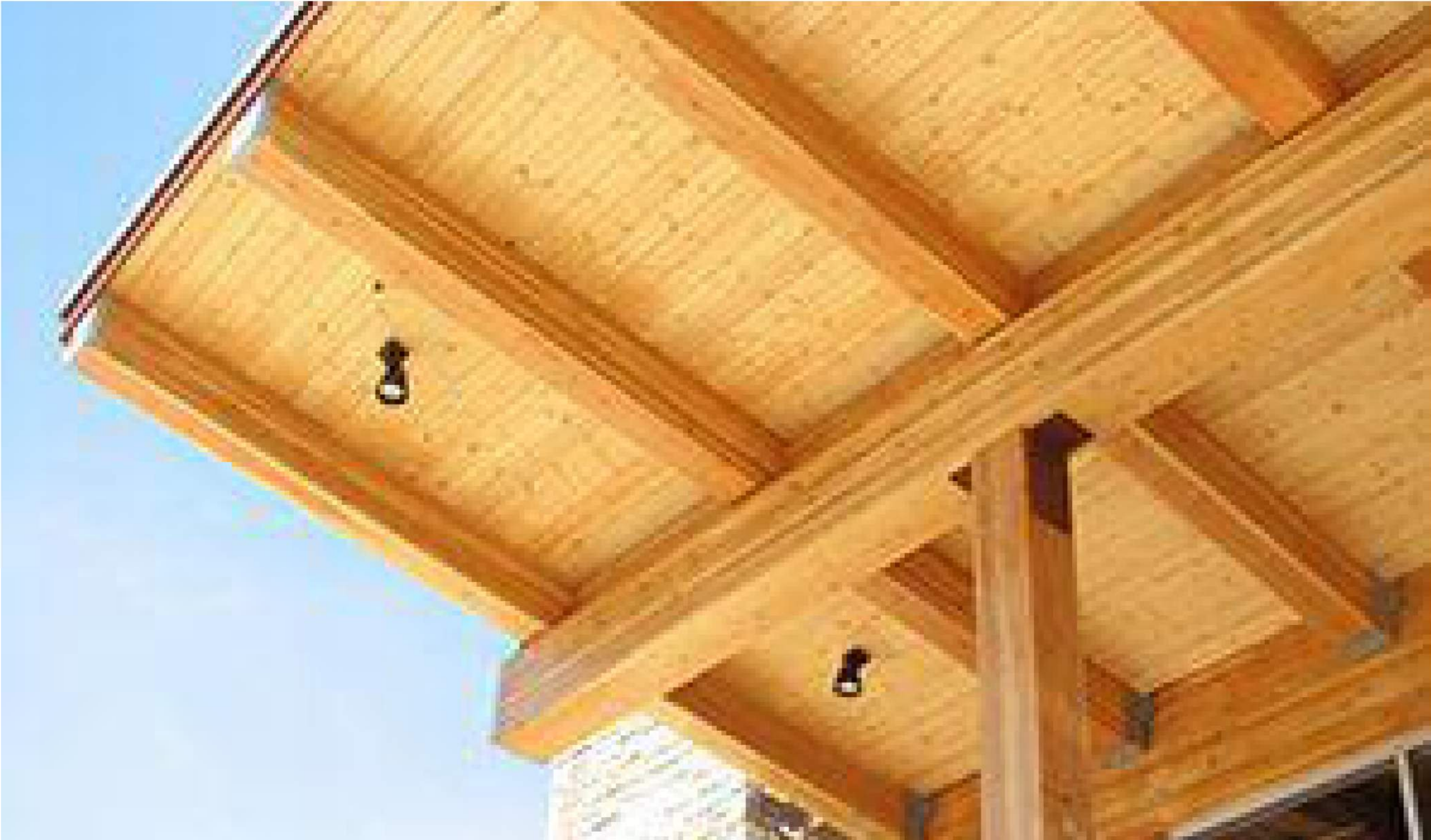
GLU-LAMINATED BEAMS AND COLUMNS
