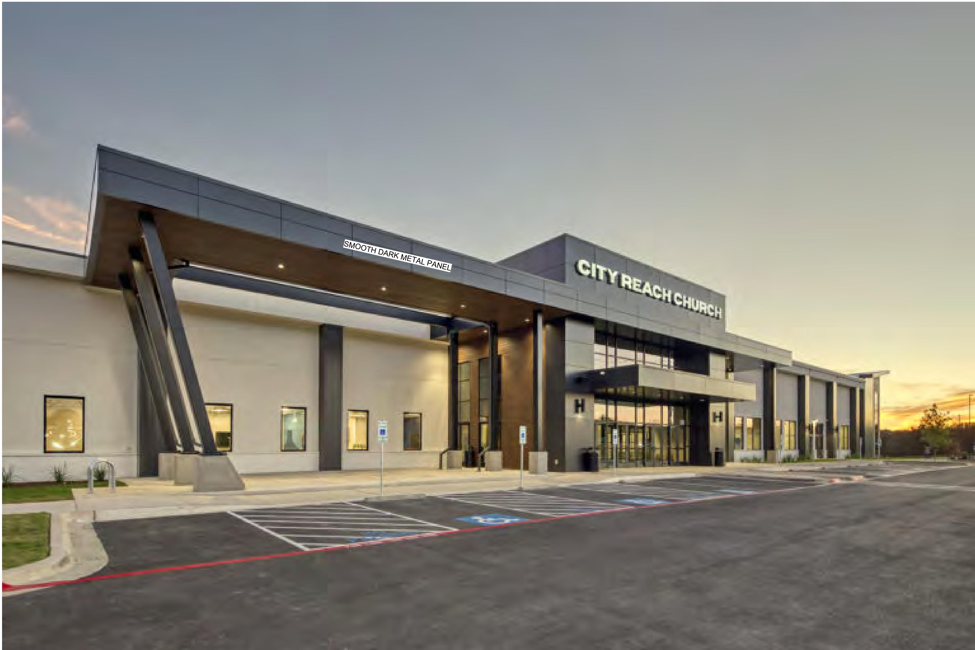
CITY REACH CHURCH | CEDAR PARK, TX
