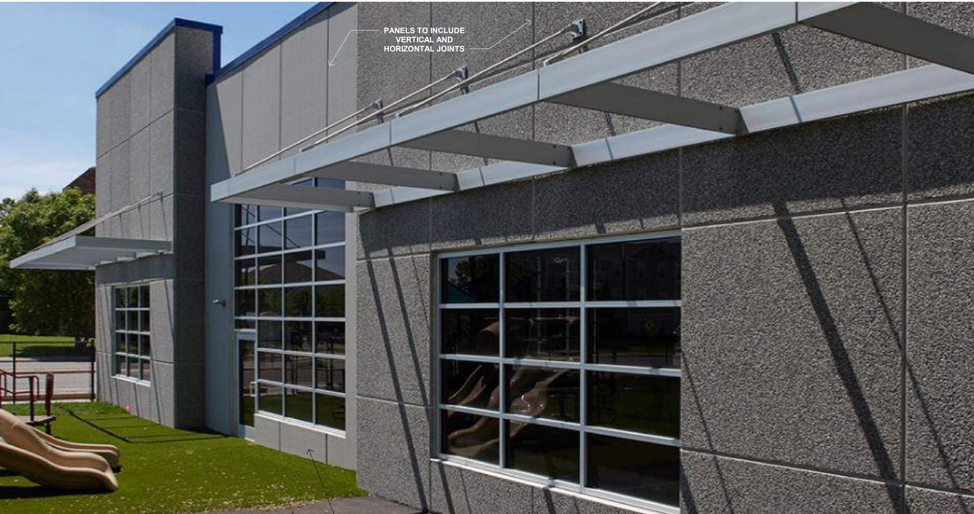
ARCHITECTURAL PRECAST PANELS
