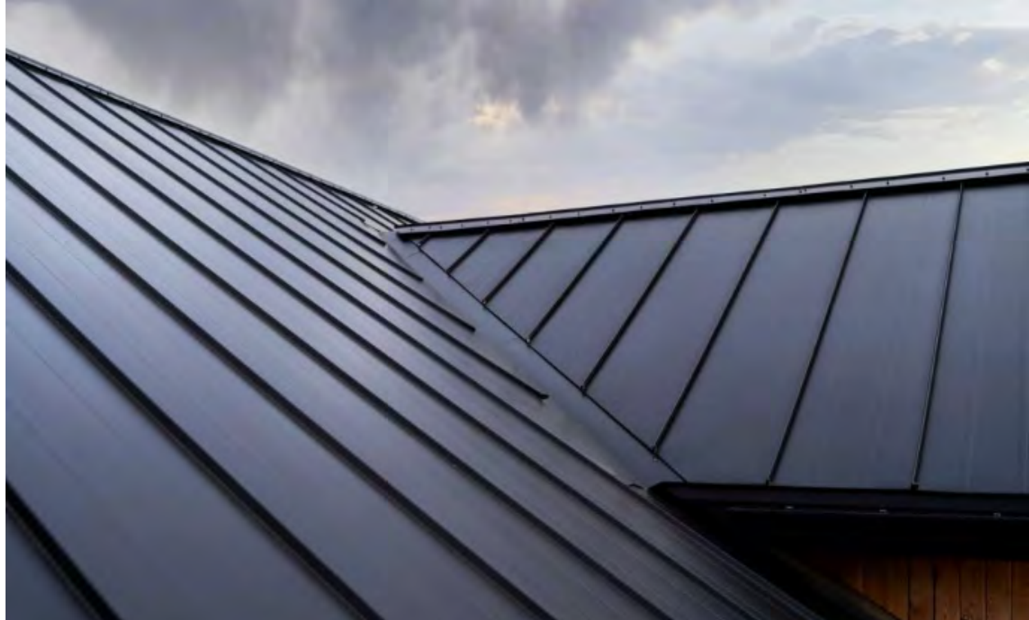
STANDING SEAM METAL ROOF EXAMPLE
