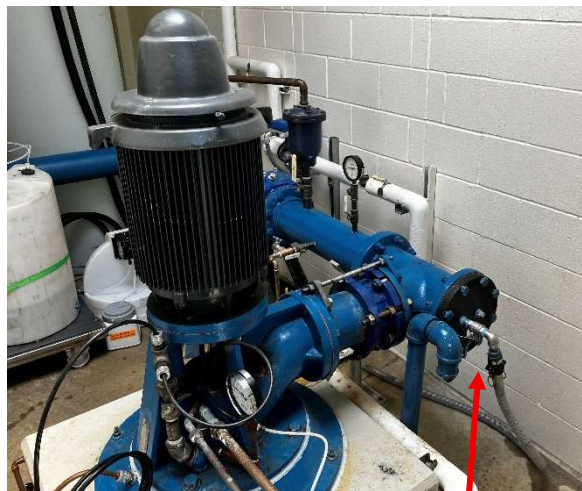
Figure 2. Pilot Feed Connection
