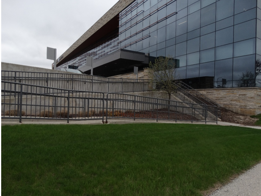
Existing ramp near private path – Looking east
