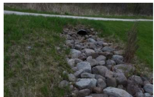
One of many existing culvert outfalls at ponds
