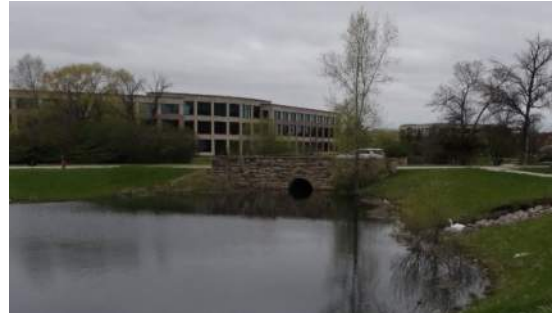
Structure along south Riverwood Drive
