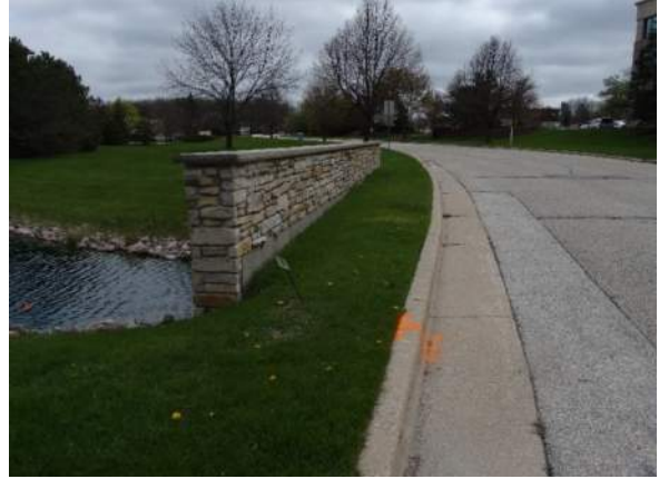
Existing structure, terrace, and parapet at roadway
