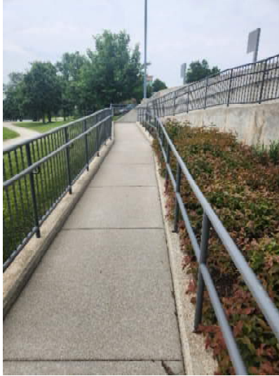
Existing Ramp at west side of ProHealth
