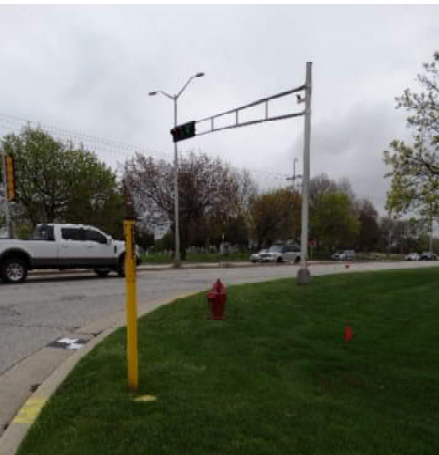
Existing gas, water, fiber, and signals at the Riverwood Drive south and Pewaukee Road
