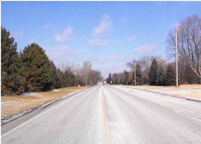
Looking north from Glenwood Lane
