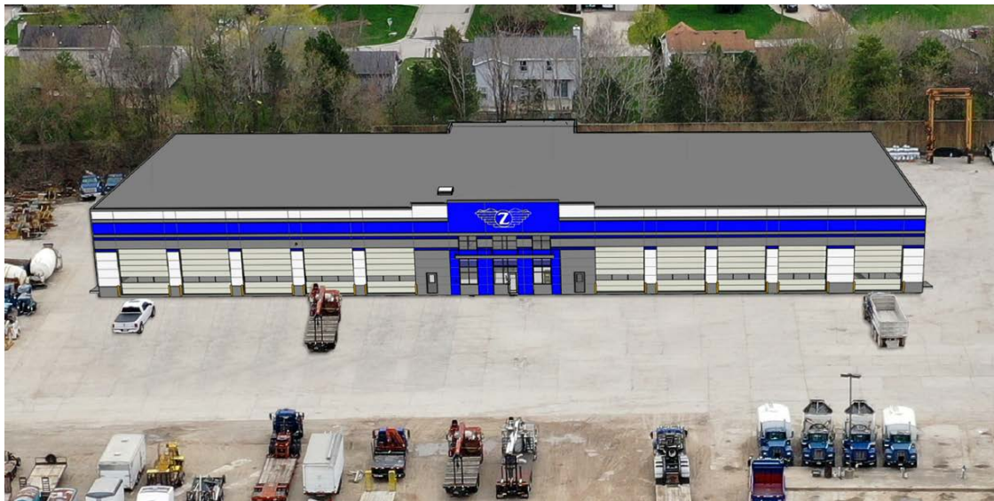
Zignego Corporation W226N2940, W226N2966, and W226N2974 Duplainville Road 24,800 square foot repair facility
