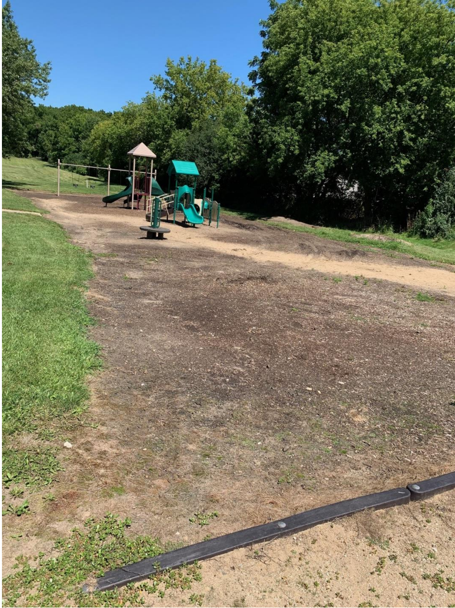
Existing conditions of removed playground structure that was unsafe (removed 2019)
