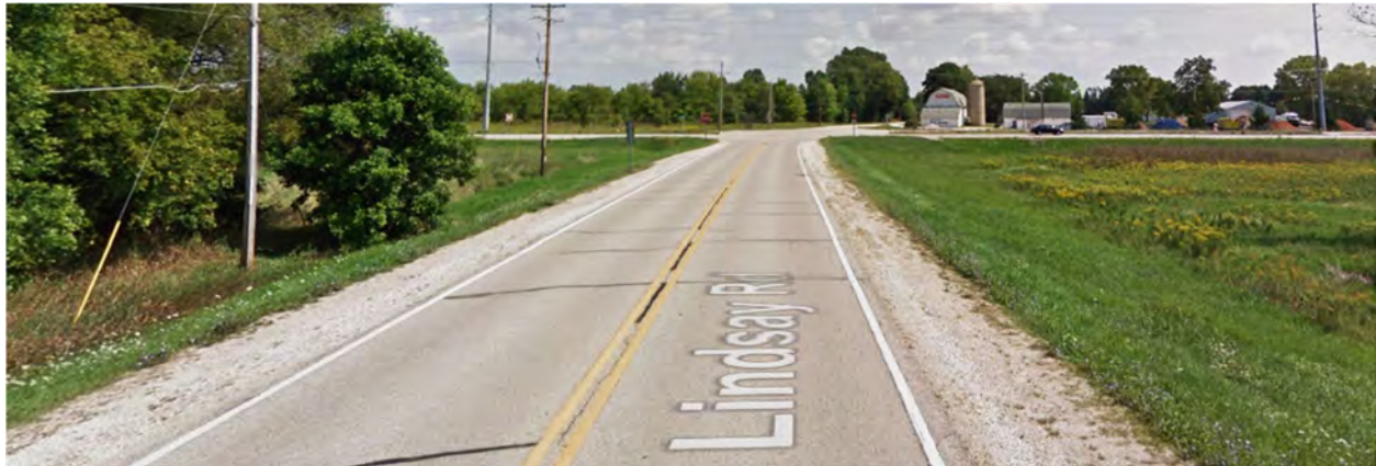
Figure B3 Lindsay Road Looking East Approaching CTH F
